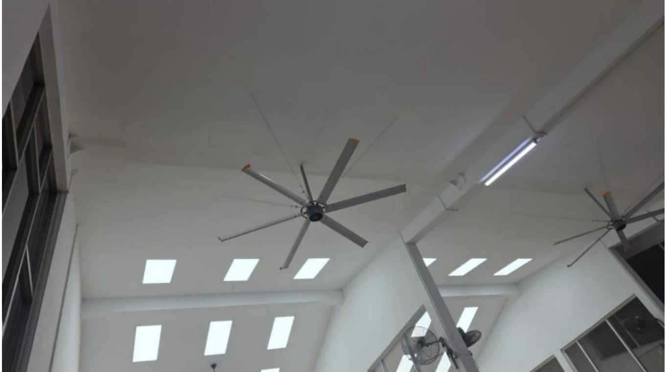
After: the installed HVLS fans.
